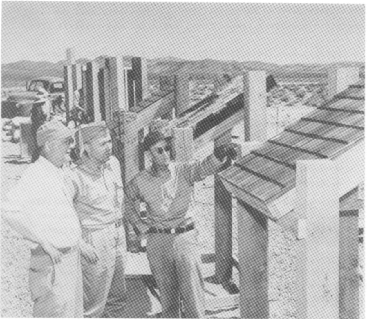
Figure 4-4: PROJECT 8.5 PERSONNEL EXAMINE ROOFING MATERIALS TO DETERMINE THE THERMAL EFFECTS PRODUCED BY A NUCLEAR DETONATION
