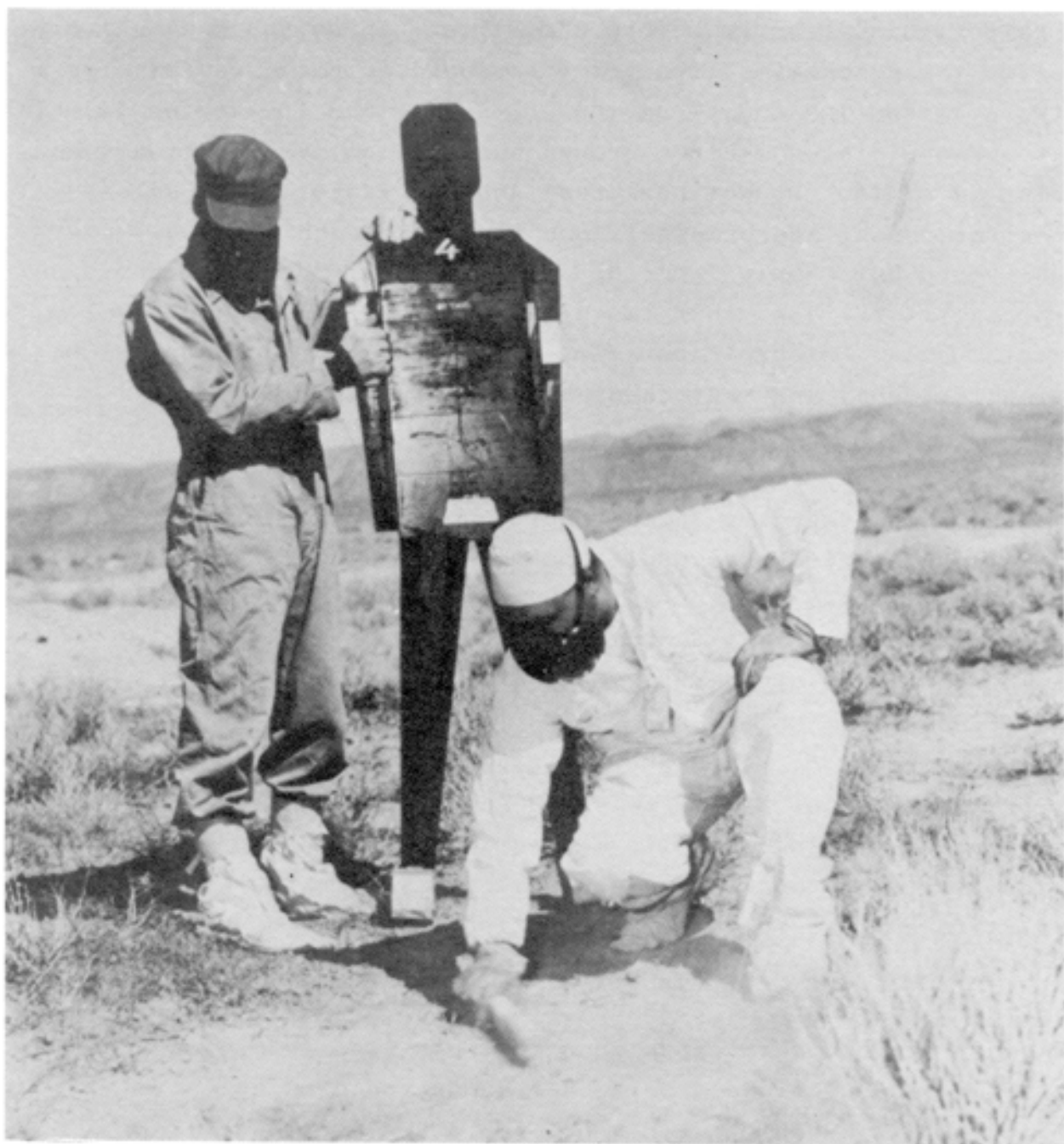
Figure 2-3: PROJECT 2.6 PERSONNEL PLACE MANNEQUIN TO COLLECT DATA ON RADIATION AND ITS CONTRIBUTION TO BODY DOSE
