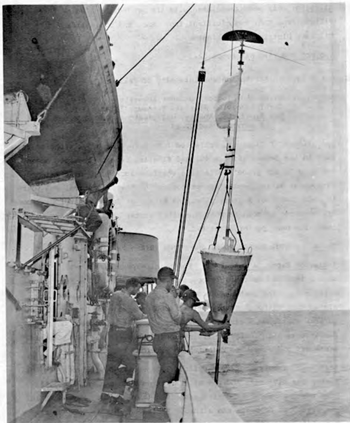
Figure 45. Placement of anchored fallout collector buoys, CASTLE.
