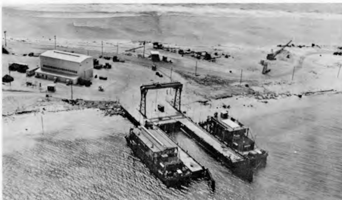
Figure 7. Assembly area on southern tip of Parry looking south, CASTLE.
