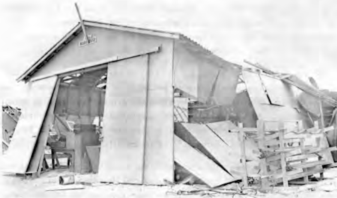
Figure 56. CASTLE, BRAVO blast damage to Eneman Island building.
