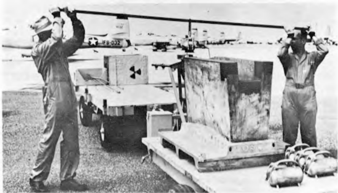
Figure 33. Lifting pig containing filter paper, CASTLE.
