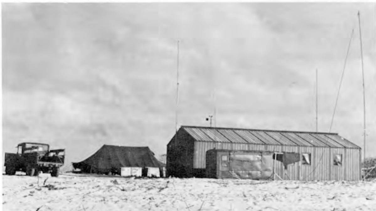
Figure 64. Photo of Rongerik installation, CASTLE.
